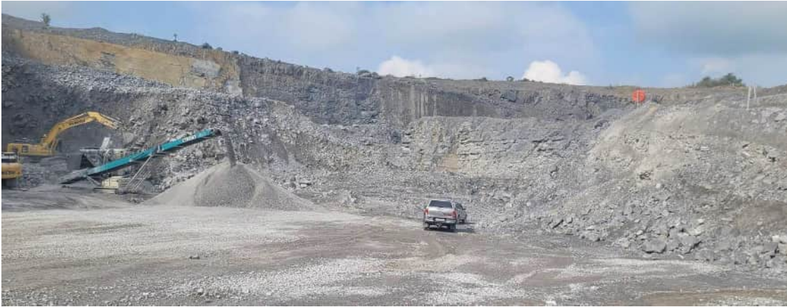
Plate 4: August 2026 – View from Southwest Corner of Quarry – above Sump / Infiltration Area looking East
